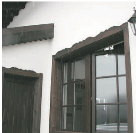
All windows are double glazed with wood surrounds.
