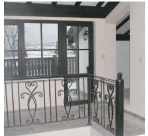
Upper landing with access to the balcony.
