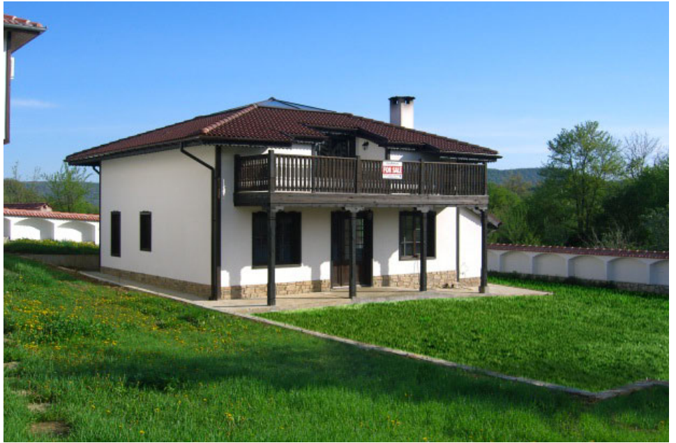
The finished cottage.
